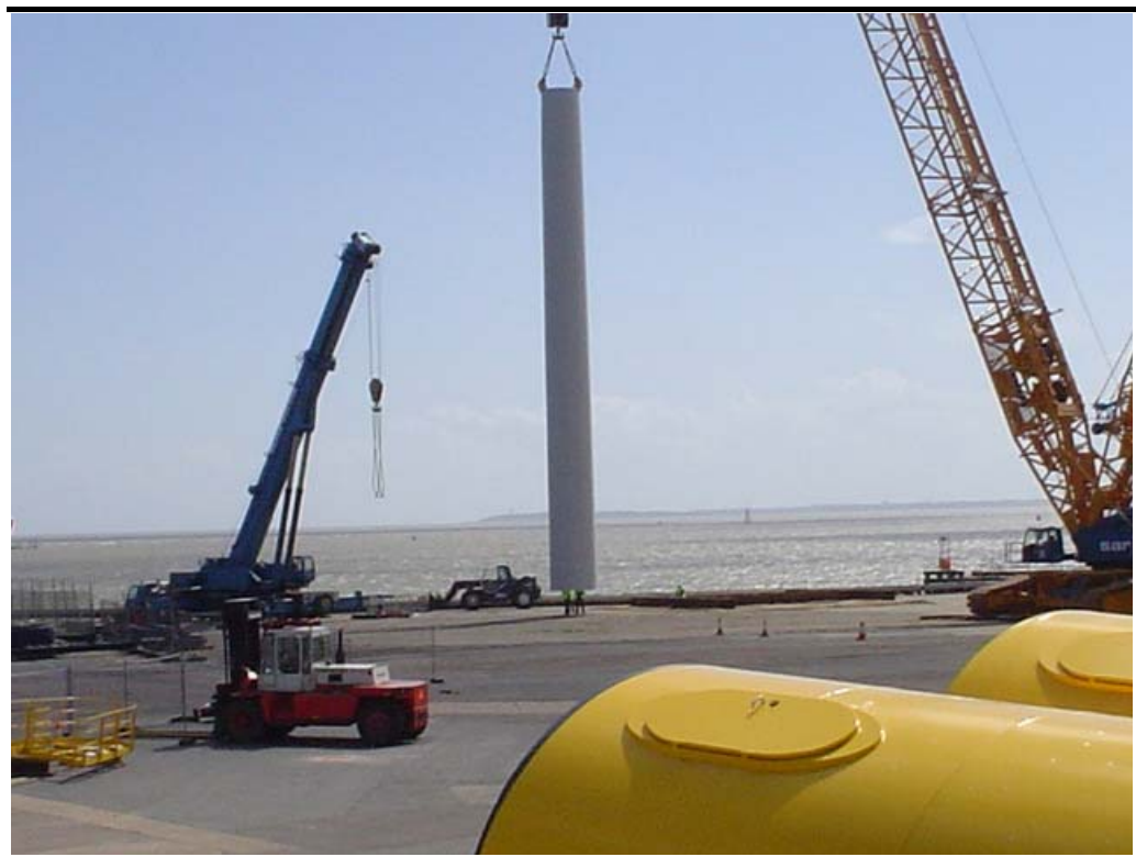
Figure 11.21 Typical Mast Assembly 2
